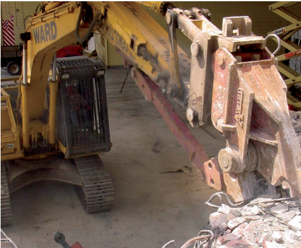
IMAGES: (D) Removing suspended floors: (E) & (F) Close view of Concrete Shear Jaw
